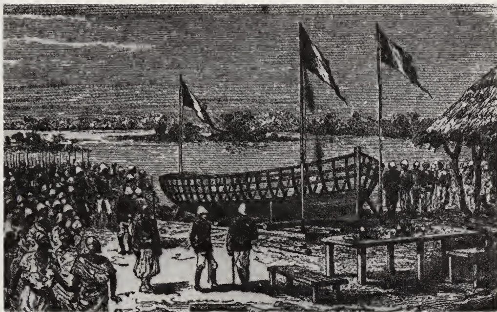
A French gunboat being constructed on the Niger
