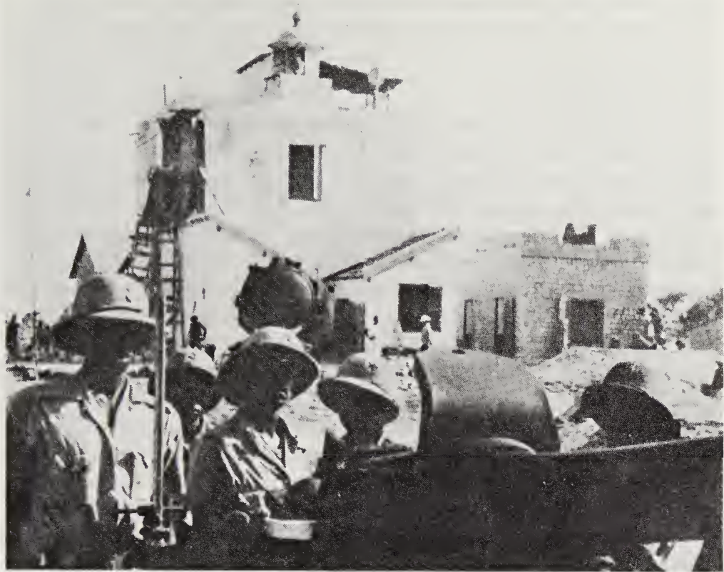
Batteries at Dakar being manned by African soldiers
